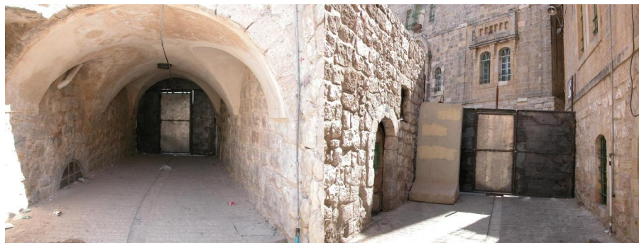
Figure 2-21: New iron gates placed to close Al-Qasaba from the eastern direction. Source: HRC, 2005
