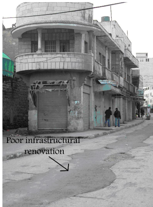
Figure 2-14: Example of Infrastructural restoration done on a small scale
